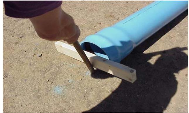
Manual assembly of small diameter pipe may be accomplished using only manual force. The block and bar method of assembly is recommended for larger diameter requiring a greater insertion force. This method allows workman the ability to judge the amount of force and determine if undue resistance exists. Be sure belled end lengths are properly braced to avoid over-insertion of previous joint.
