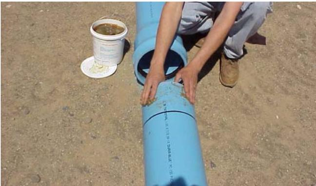
Lubricant used must be approved for potable water (PW) service. Use lubricant supplied with pipe or recommended by pipe manufacturer.
