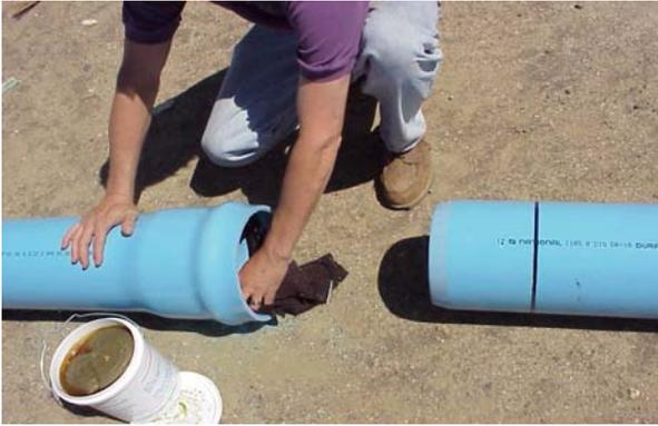
It is important when assembling PVC pipe cut in the field the spigot end should be inspected to ensure that the cut is perpendicular to the pipe's longitudinal axis. Edges should be deburred and beveled and the insertion line reapplied. The integral bell and spigot must be cleared of dirt and foreign material with a clean rag. Spigot end should be cleaned beyond insertion line.
